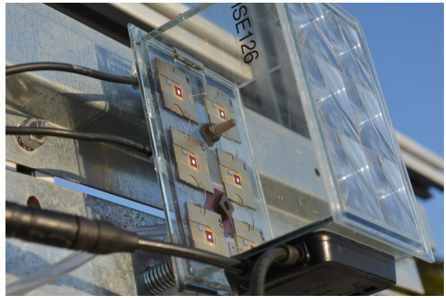
Fig. 2. One of the completed test modules installed on the 2AP tracker.
